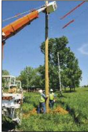
At top right is the new substation switch house being delivered for set-up on the prepared site. Currently, the house is being wired with the needed communication and control devices that will automate the substation. Above, workers install a new pole in Elora as part of line upgrades. At bottom right is the first 161-kilovolt transformer delivered to Park City Substation on April 21.
