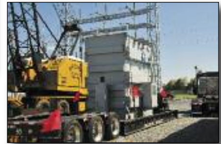
At top right is the new substation switch house being delivered for set-up on the prepared site. Currently, the house is being wired with the needed communication and control devices that will automate the substation. Above, workers install a new pole in Elora as part of line upgrades. At bottom right is the first 161-kilovolt transformer delivered to Park City Substation on April 21.
