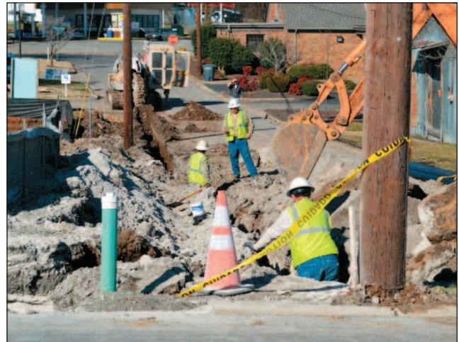
*As with any new utility construction, FPU's own water, electric and telecom crews will install utilities to the new administration building. Here, water crews dig the trench for the a new 6-inch water line.*
